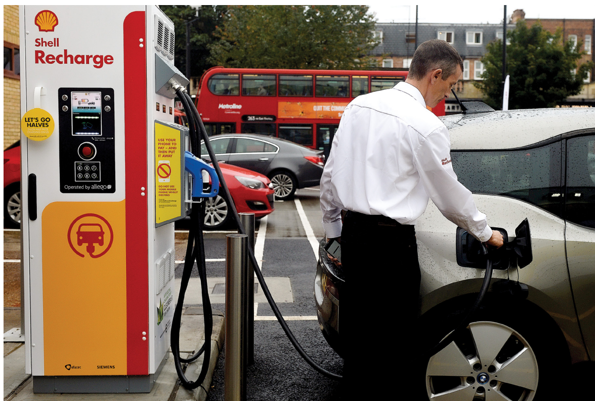
A member of staff charges an electric car at the Holloway Road Shell station where Shell is launching its first fast electric vehicle charging station in London, United Kingdom, October 18, 2017. REUTERS/Mary Turner
